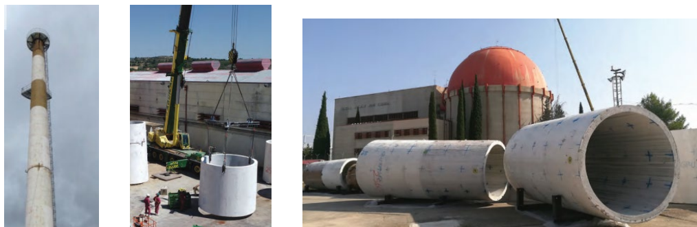
Segmentation of the José Cabrera's chimney for radioactive gaseous emissions
