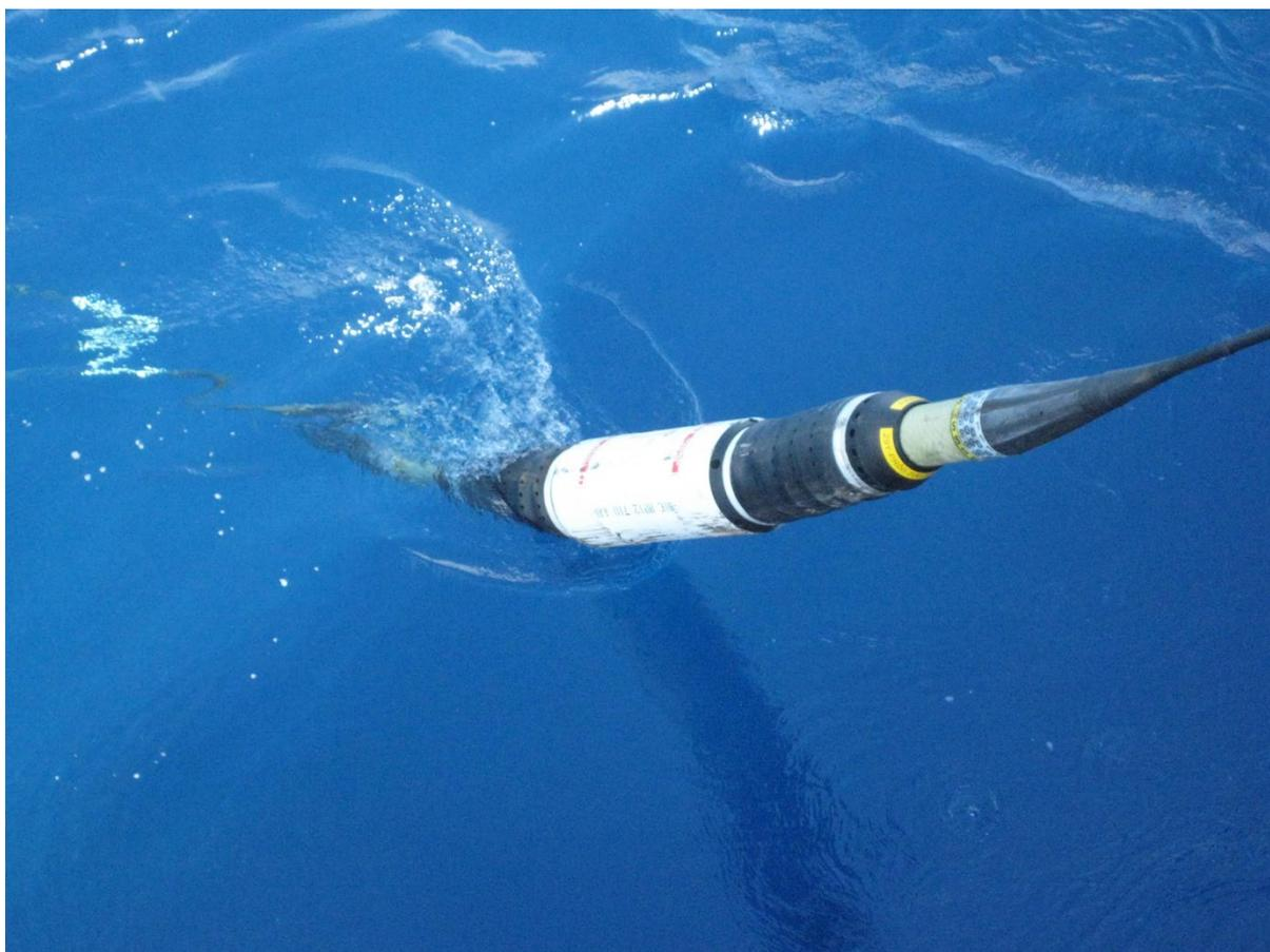
Figure 2 A repeater being deployed from a cable ship. Image courtesy of Glenn Lipsham, ESCA.
