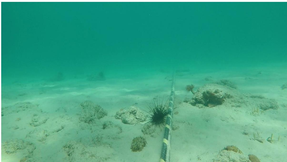
*Figure 1 Surface laid fibre optic telecommunications cable (approx. 24mm diameter). Image courtesy of Glenn Lipsham, ESCA.*
