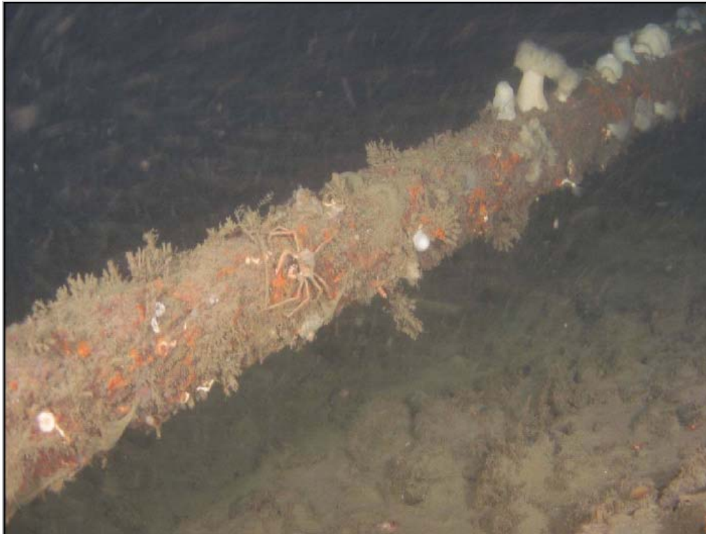
Figure 4.25 Subsea power cable, in place for approximately 50 years, covered with sessile encrusting organisms at Vancouver Island (BCTC 2006).
