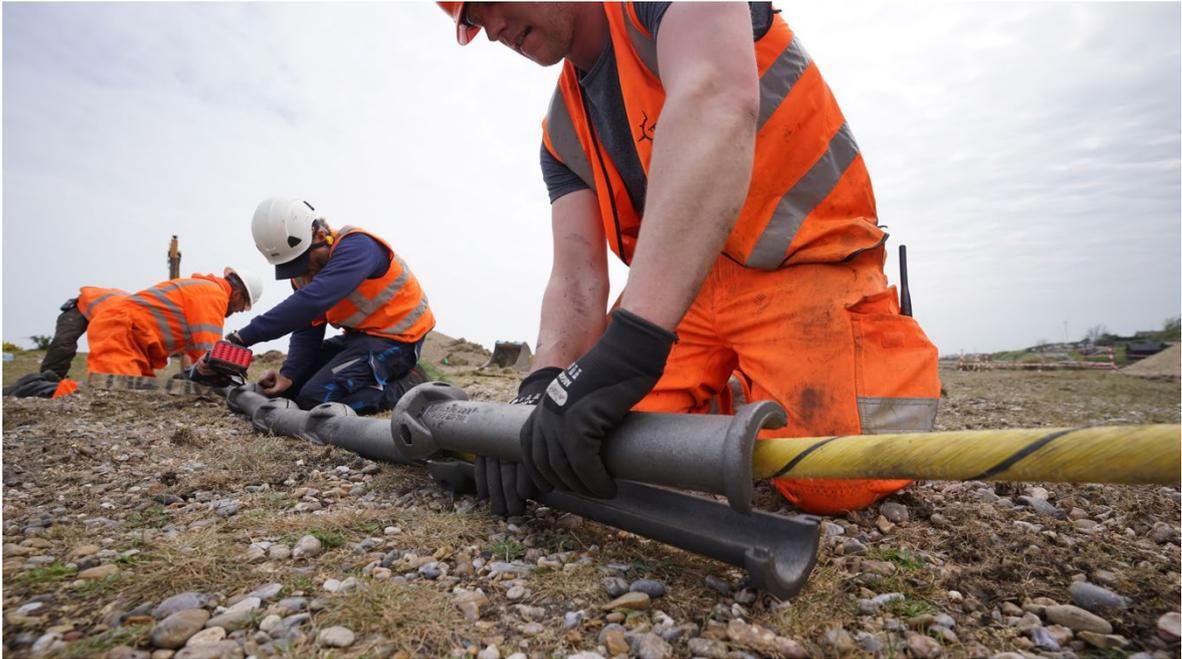
*Figure 9 Articulated Pipe being applied to telecommunications cable. Photo courtesy of Pelagian Ltd.*
