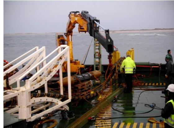
Figure 208 A Cable Joint In An HVDC Power Cable : Image D. Sinclair TenneT Offshore GmbH.
