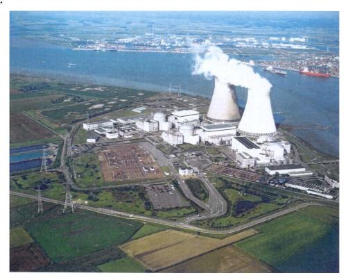
**Origin**: there are 4 reactors and in each reactor building there are 3 kinds of liquid wastes: recyclable waste waters (leakages from primary circuit) from the controlled areas called "primary waters", non-recyclable waste waters (floor, laundry, lavatory, chemical, "demineralisation effluents" from steam generators) from the controlled areas and non-recyclable waste waters (floor, regeneration effluents from machinery, ...) coming from other non-controlled areas.
