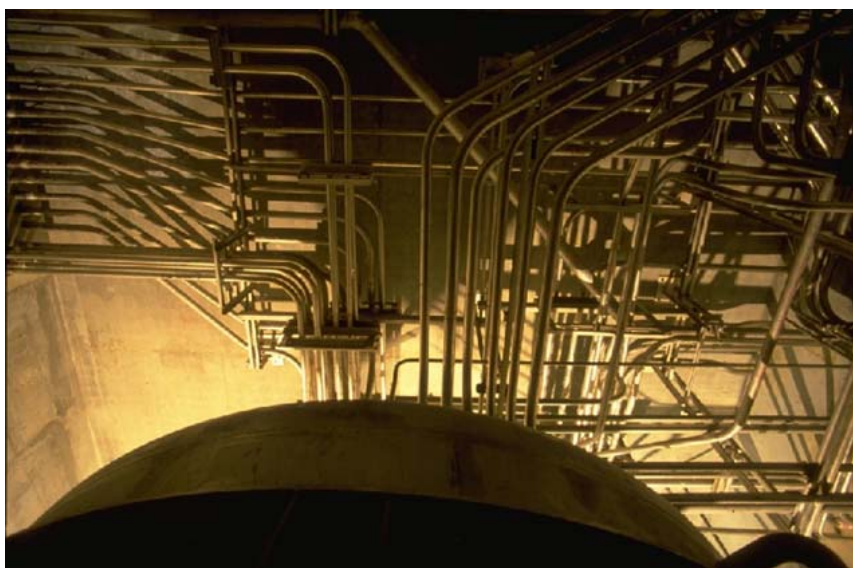
The piping above an effluent tank
