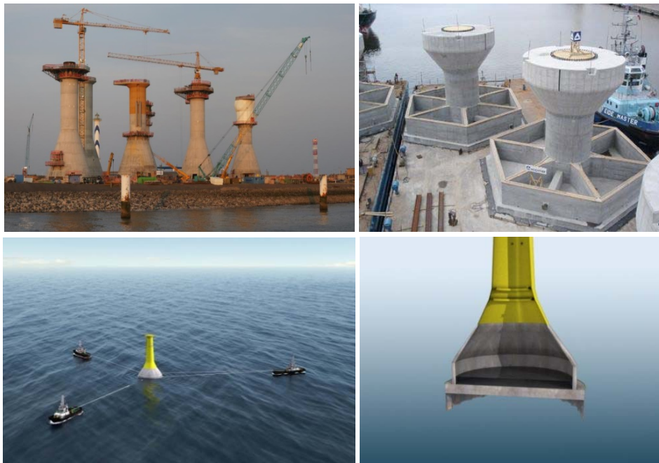
Figure 8: Above: Gravity base foundations of the OWFs Thornton Bank ( left , source: Wikimedia Commons) and Lillgrund ( right , source: Freisen 2010). Below: Seatower CraneFree gravity base foundation. The bottle shaped foundation is towed to the site and positioned ( left ). Steel skirts at the bottom ( right ) provide additional stability (source: Seatower 2013)
