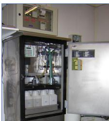
TELERAD also has 6 stations (BCI) in the release channels of the nuclear power plants which continuously measure the gamma radioactivity of the releases: one in the release channel and one upstream/downstream of the nuclear power plant of Doel and three in the release channels of the nuclear power plant of Tihange. These stations allow to monitor the liquid discharges from the electricity producers with close attention.
