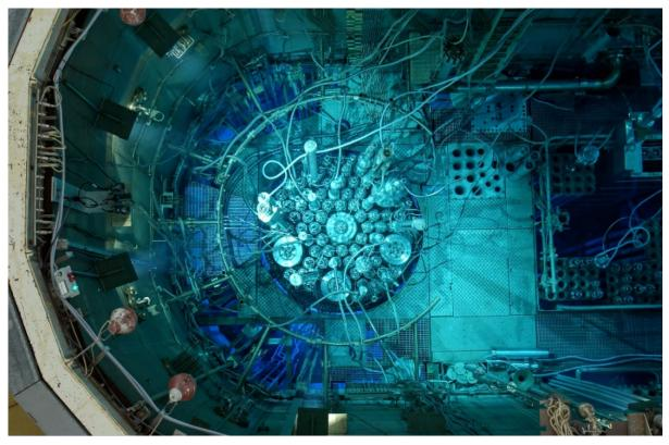
The BR2 is a heterogeneous thermal high flux test reactor, designed in 1957 for SCKCEN by NDA [Nuclear Development Corporation of America - White Plains (NY - USA)]. It is also built and located on the site of the SCKCEN in Mol.
